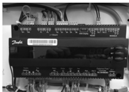
Picture 3: Normal wiring
