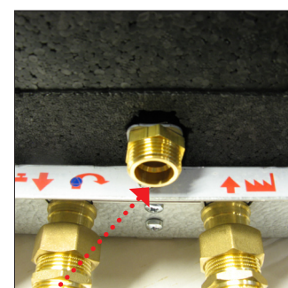
Circulation pipe connection
