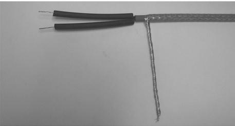
4. Crimp tube 4/1, L=70 mm is pulled on to the two stripped wires.
