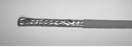
1. The heating cable is stripped over a length of 90 mm.
