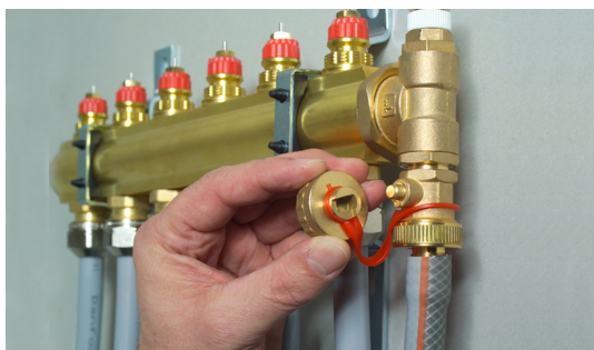
Fig. 5: Shut off main supply and return ball valves. Heating circuits are individually flushed via fill and drain valves mounted on respectively supply and return manifold.
