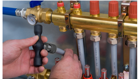
Fig. 2: Centre pipe and bevel with bevelling tool - 2 mm all round bevel on inner pipe.
